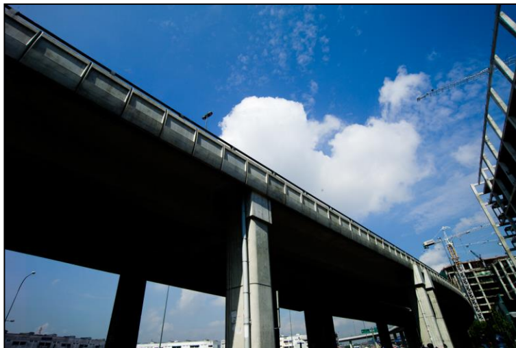
Figure 2: A construction site of fly-over ramp located near Seri Kembangan, Selangor, Malaysia.
